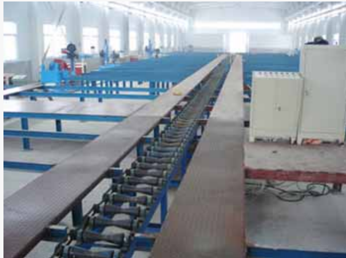
Pipe Logistics Automatic Transport System
