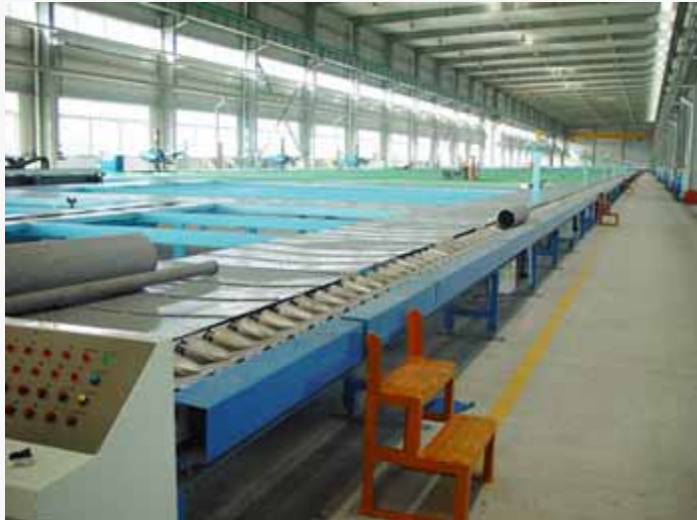
Pipe Logistics Automatic Transport System
