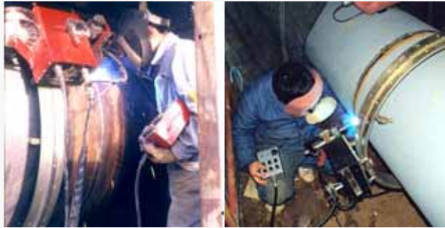
Piping All-position Automatic Welding Machine(FCAW/GMAW)
