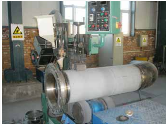
Piping Prefabrication Automatic Welding Machine(SAW)
