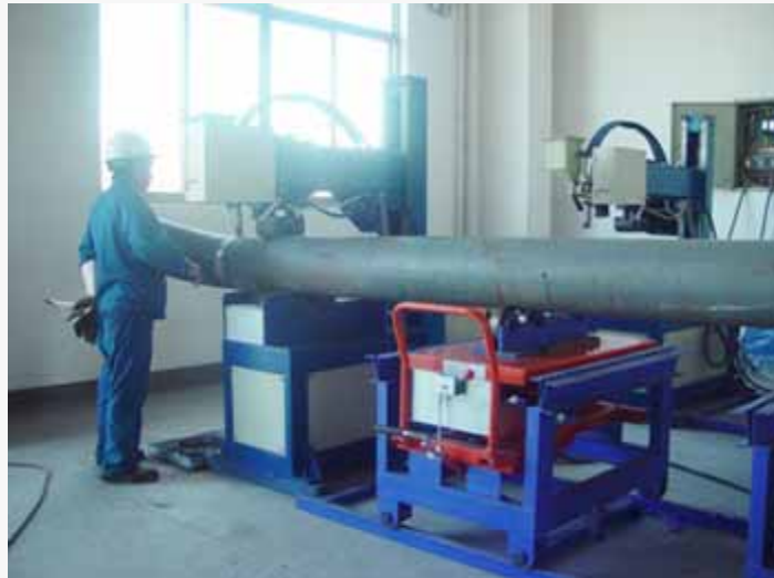
Piping Prefabrication Automatic Welding Machine(SAW)
