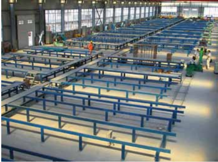
Piping Prefabrication Production Line (Fixed Type)
