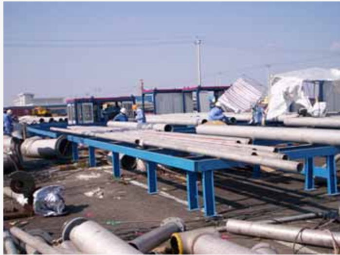
Tansportable Piping Prefabrication Production Line
