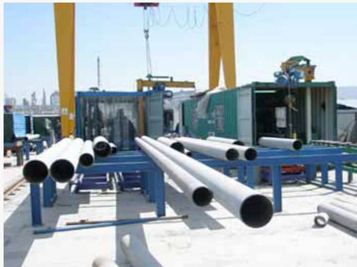
Tansportable Piping Prefabrication Production Line
